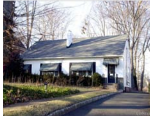
For Lease - 3,100 sf 23 Village Green Road Madison, NJ
