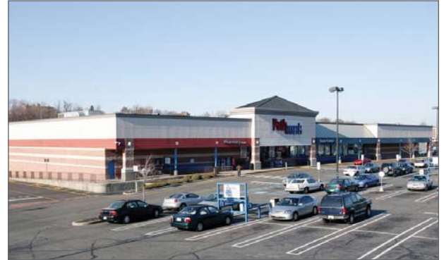
175 Passaic Avenue, Kearny
