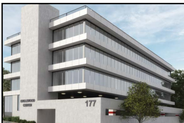
177 N. Dean Street Englewood, NJ 4,756-8,150 sf for lease
