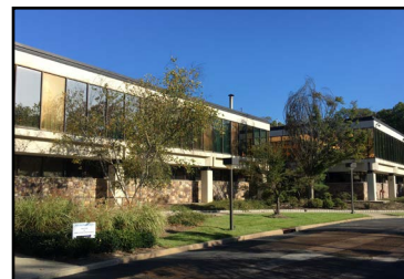
1700 Valley Road Wayne, NJ 69,163± sf for lease
