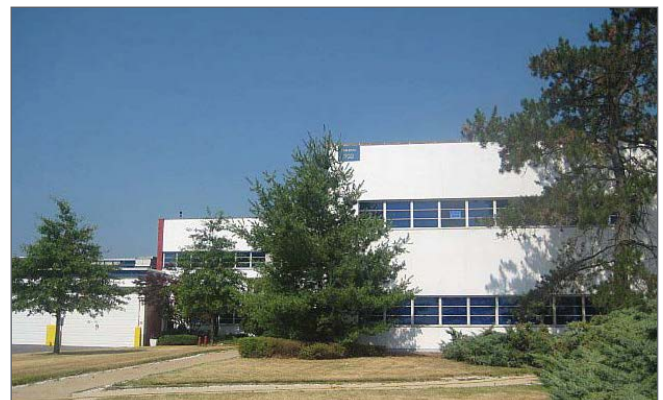
2300 Route 1, North Brunswick
