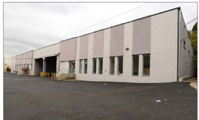
585 Industrial Road, Carlstadt
