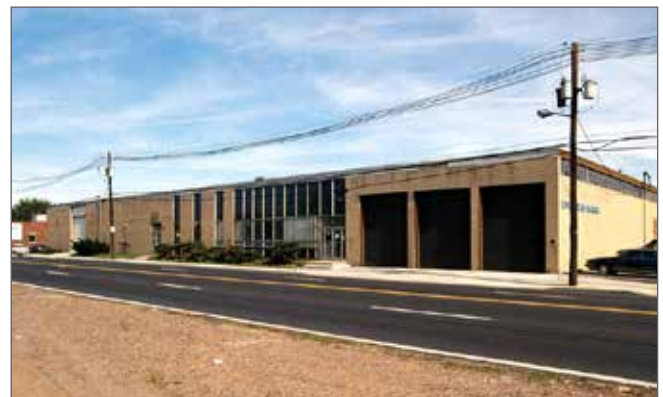
4000 Westside Avenue, North Bergen
