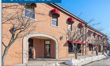
201 Rock Road Glen Rock, NJ 2,180 sf
