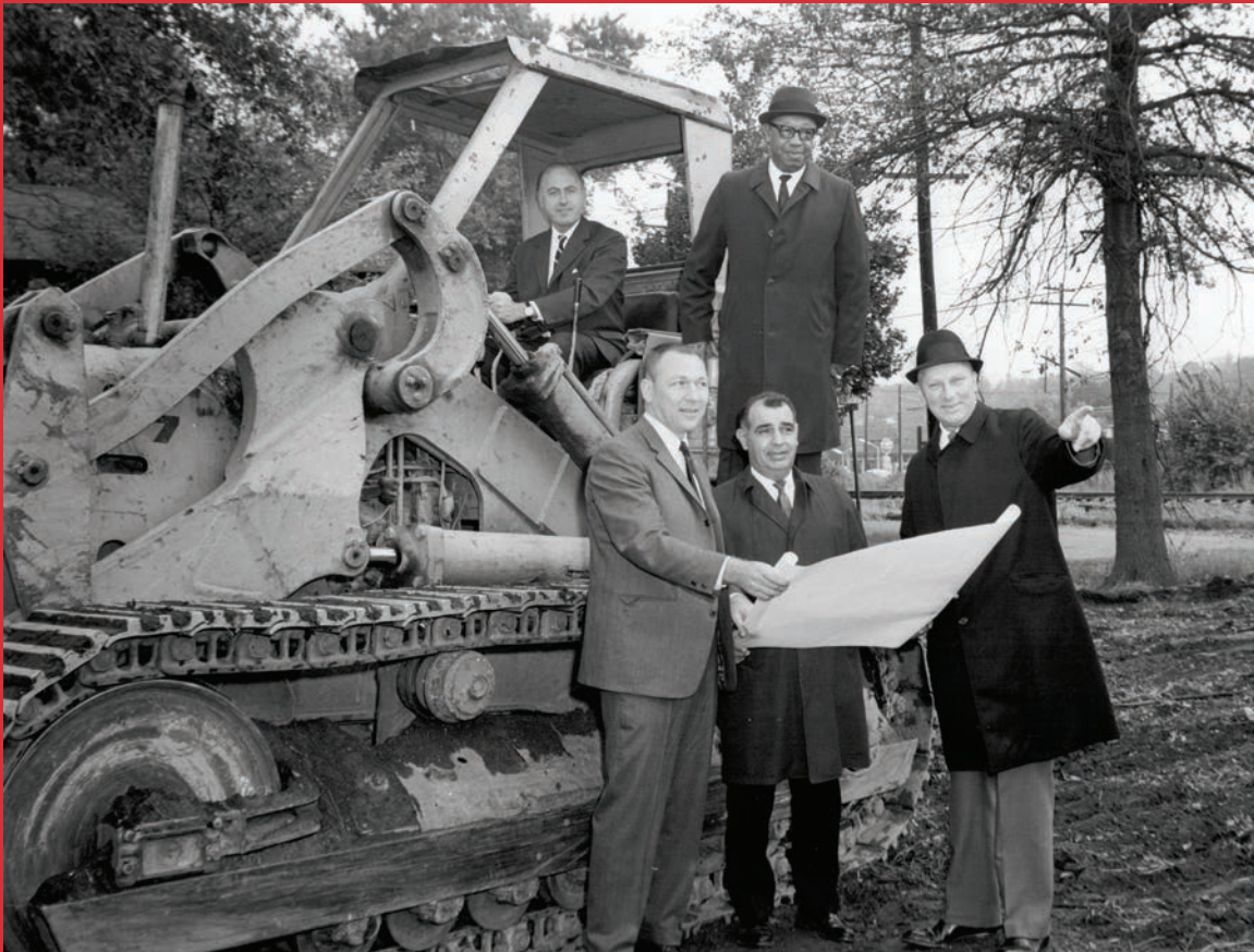
1962- Building the Englewood post office, where it stands today. Peter O. Hanson, standing on far left.
