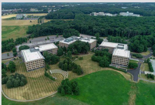
78,391 SF 777 Scudders Mill Road Plainsboro
