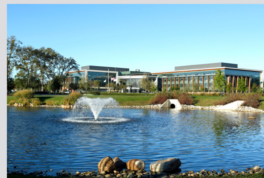
72,326 SF One CommVault Way Fort Monmouth*
